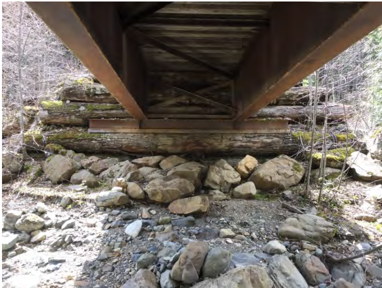
Left Bank Abutment when facing downstream
