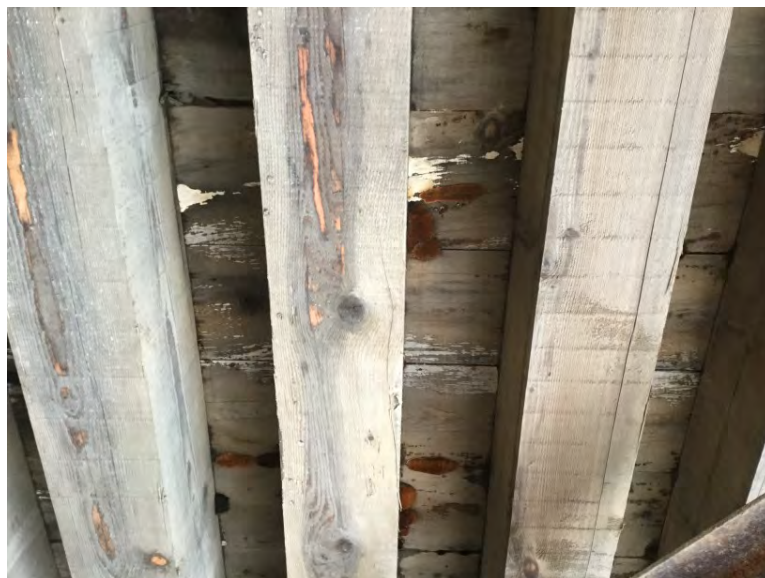
Subdeck condition at right abutment
