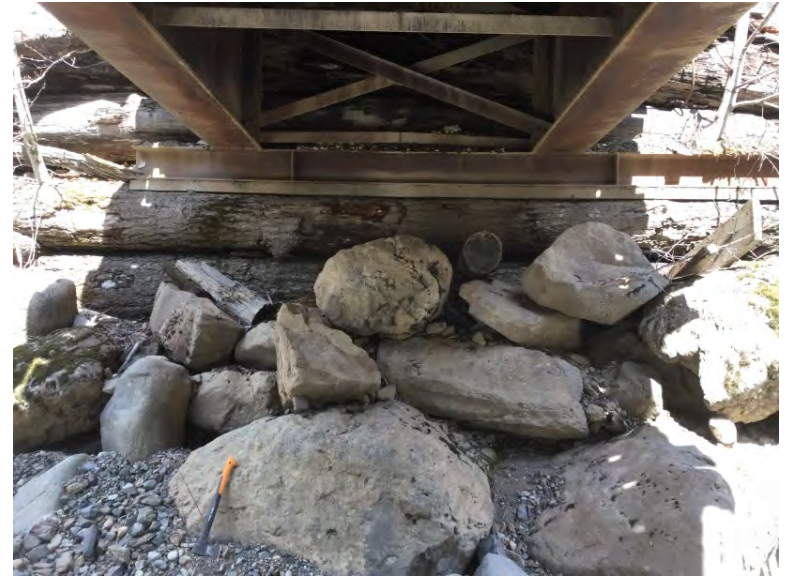
Right Bank Abutment when facing downstream
