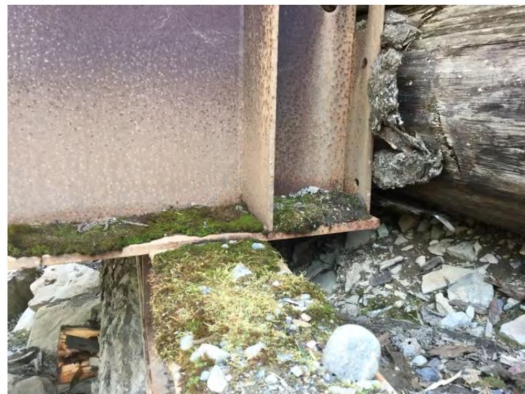
Bearing at downstream left bank
