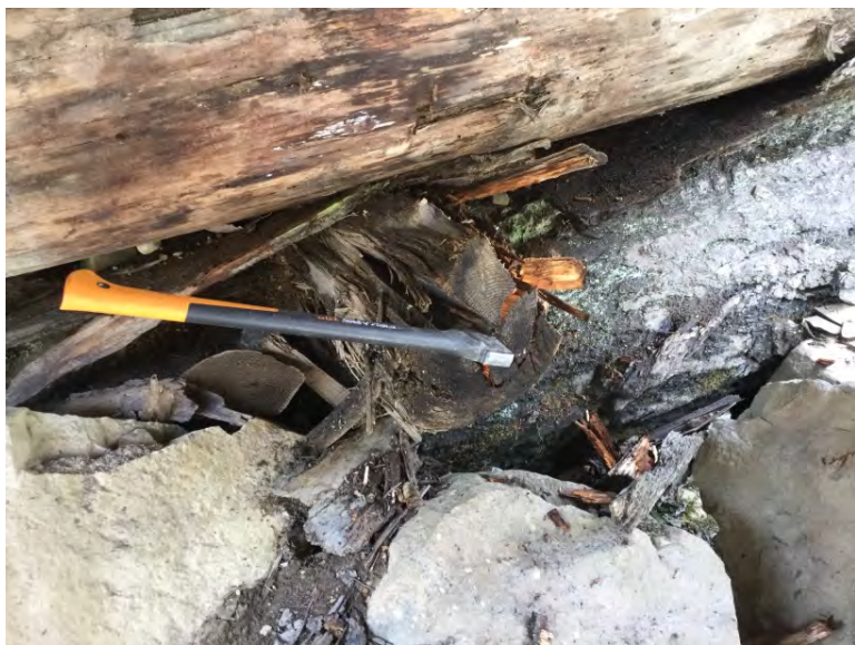
Tieback condition at left bank
