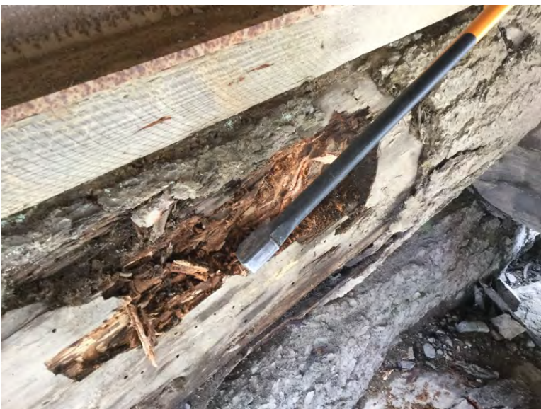
Top face log condition at right bank abutment
